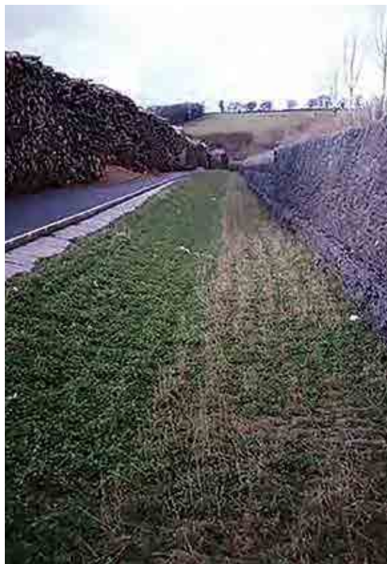
Figure 17.6 Swale with vertical side (courtesy EPG Limited)
