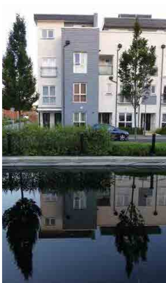
Figure 5.9 Canalside living, Redhill, Surrey (courtesy Studio Engleback)
