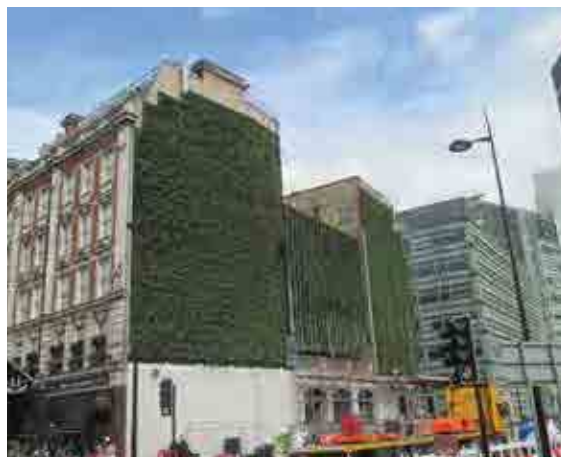
Green wall (courtesy Green Roof Consultancy)
