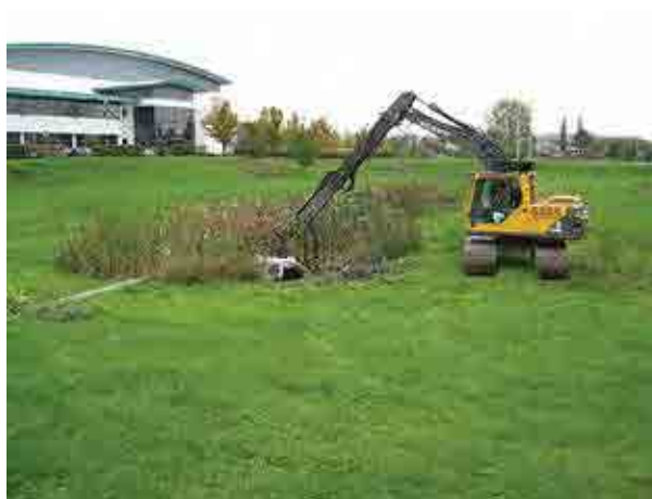
Figure 32.2 De-silting (courtesy Bedford Group of Drainage Boards)
