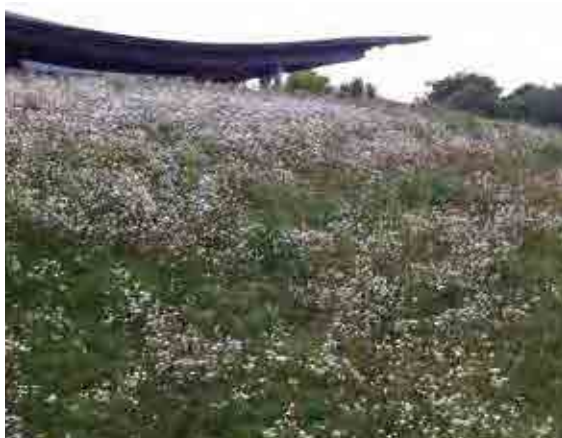
Figure 12.2 The Savill Garden extensive green roof
