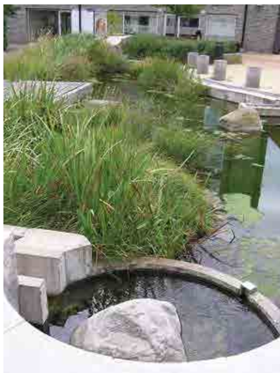
Figure 23.7 Pond with baffles and islands, Augustenborg, Sweden
