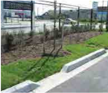
Figure 28.6 Roadside lateral inlets
