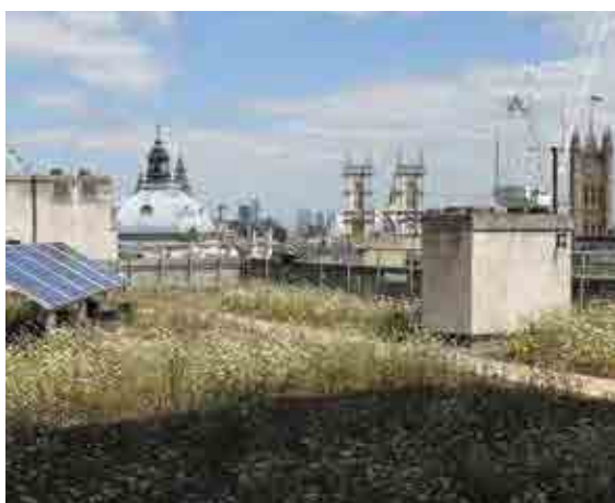
Green roof (courtesy Green Roof Consultancy)
