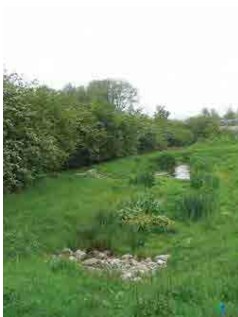
Figure 23.11 Balancing pond with marginal wetland treatment zone, Hopwood Park motorway services, M42, Worcestershire
