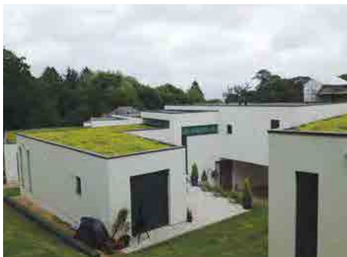
Figure 12.5 Domestic green roofing, Swansea (courtesy Sky Garden)
