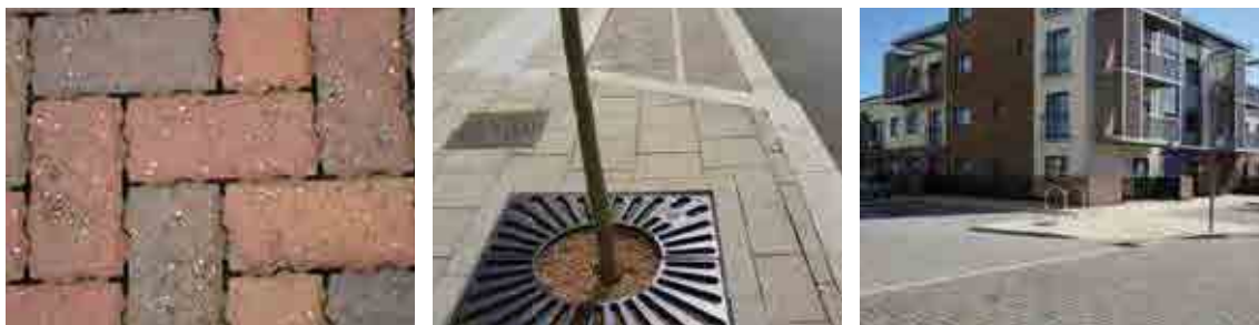
Figure 10.2 Pervious surfaces (courtesy Interpave)
