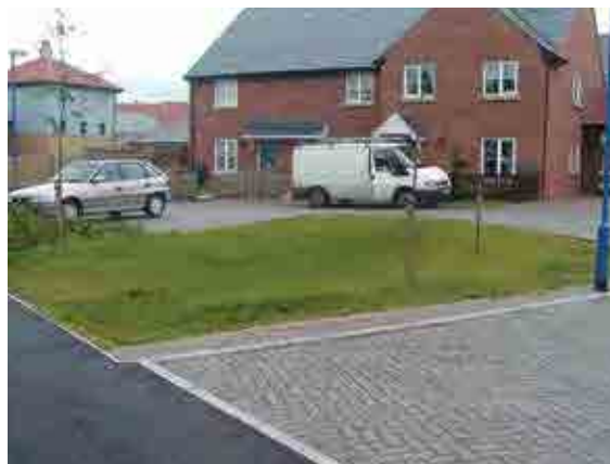
Figure 13.7 Small infiltration basin, Cambourne (courtesy Illman Young)
