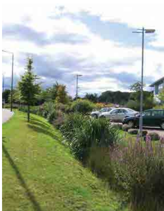
Figure 17.11 Linear wet swale, Junction 4 M8, West Lothian
