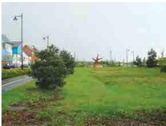
Figure 13.6 Large infiltration basins, Ipswich (courtesy Graham Fairhurst)
