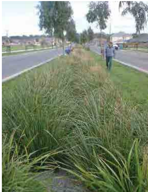
Figure 18.7 Bioretention swale (courtesy Derwent Estuary)
